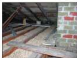
Typical vermiculite insulation in an attic
