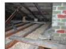
Asbestos-containing vermiculite attic insulation
