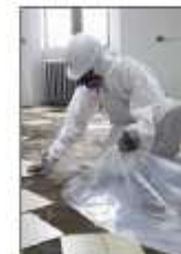
Protected worker removing asbestos flooring
