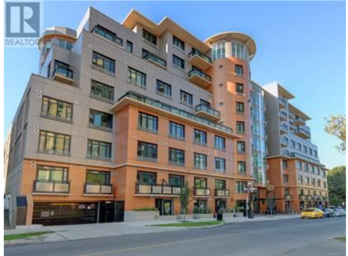
1301 Hillside Ave – Step 3
