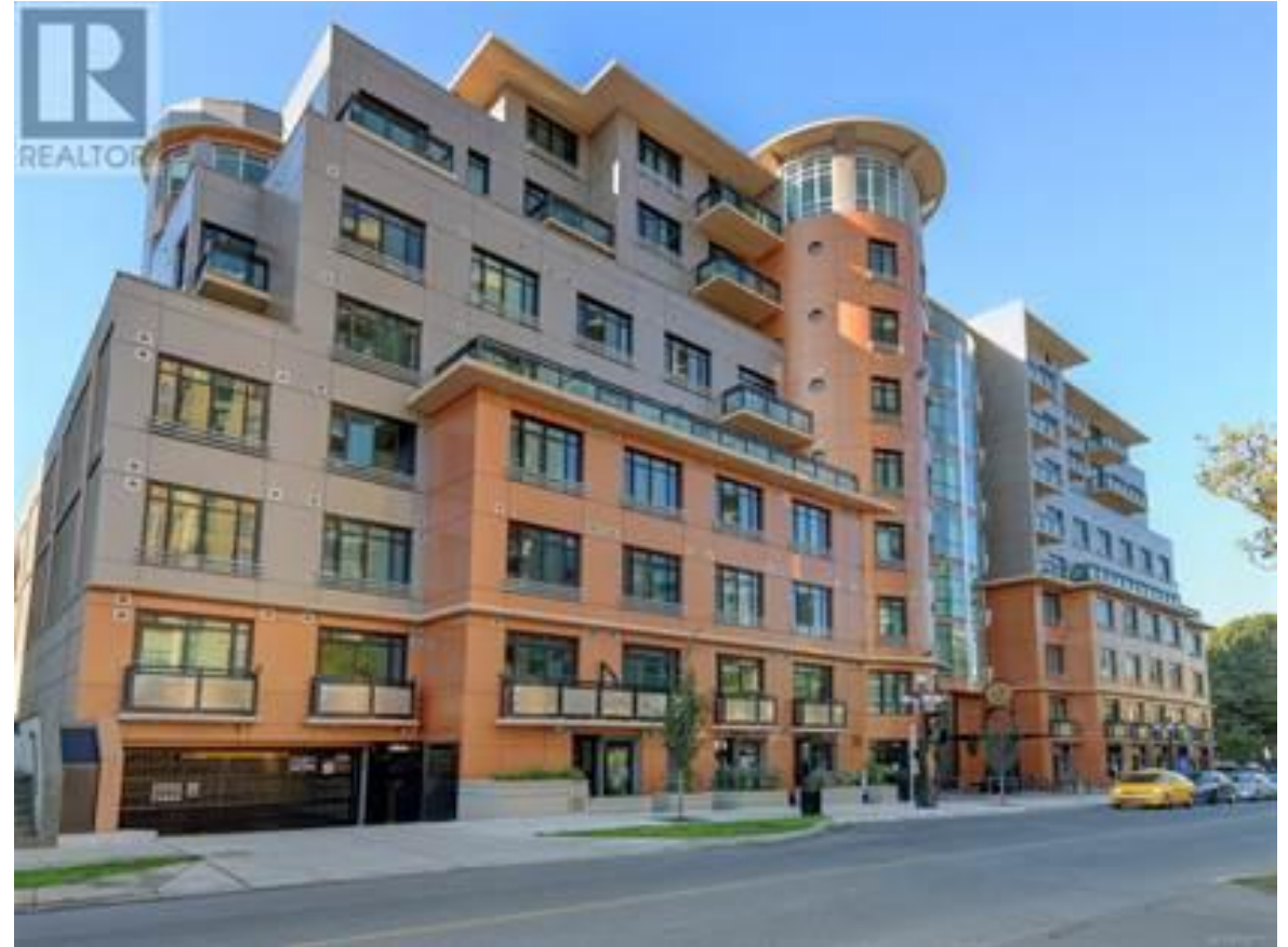
1301 Hillside Ave – Step 3
