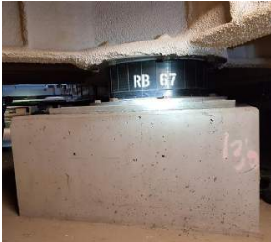
Elastomeric bearing
