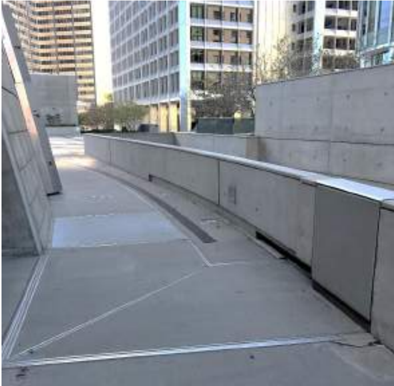
Moat cover panels
