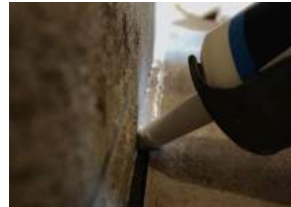
Edge Seal – Rod and Caulk
