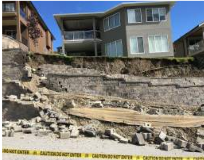
Retaining Wall Failure
