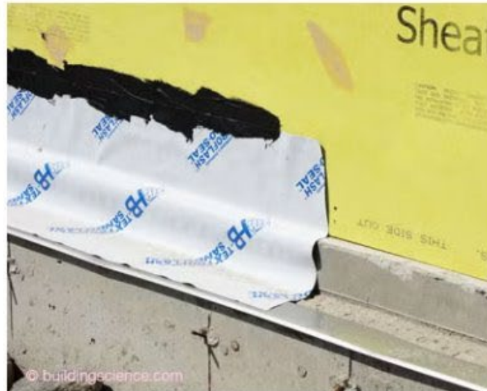
Photograph 7: Termination – This “terminate” the reverse lap thing is a big deal. A continuous bead of sealant is used to glue the top edge of the reverse lap to the underlying membrane or sheathing.
