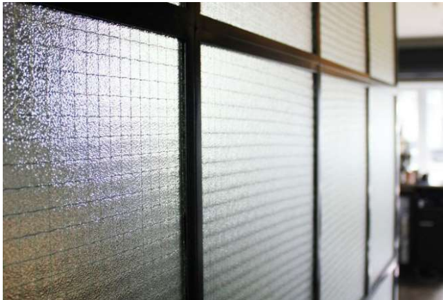
Wired Glass in Fixed Steel Frame
