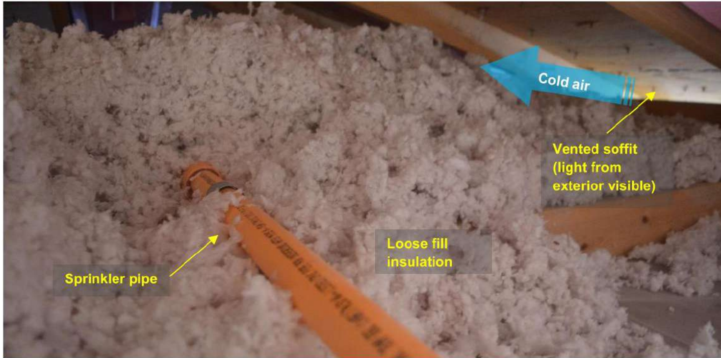
Figure 5: Loose-fill insulation without batts in some areas (including near the entrance, which had a lower roof), which buried the pipe in insulation such that it is insulated from the heated space below. Wind from the ventilated soffits can enter the attic space.
